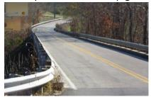
at Dutchman Creek which is also designated as a bridge. The bridges are not structurally deficient. The narrow width at the bridges is a concern particularly with recreational vehicles, trucks and farm equipment. There are several locations with high crash history. The common types of crashes from KY 1319 to KY 1633 are roadway departure crashes.
